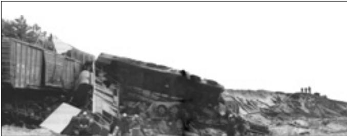
A washout is a railroader's worst nightmare — the earth simply disappears from beneath the track bed and there's nothing left to support tonnes of speeding metal. This could lead to a catastrophe with few survivors. 5
